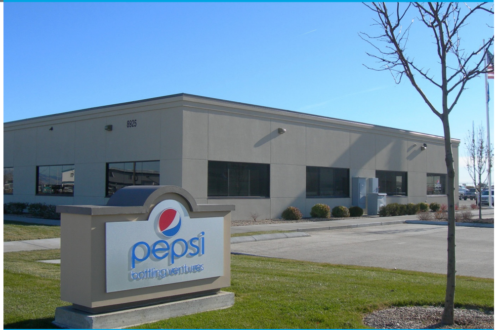
The Pepsi bottling plant in Nampa, Idaho produces and distributes carbonated soft drinks, bottled water, juices, and teas. Photo courtesy of Pepsi.
