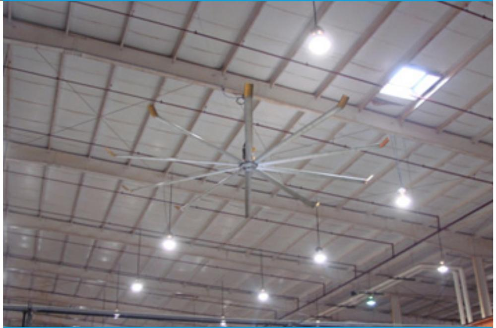
This recent SLW photo shows a destratification fan, test skylight, and new 180-watt fluorescent twin-spiral thread-in lamps that replace 400-watt probe-start metal halide.
