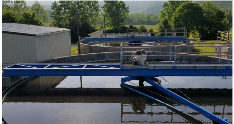
Clarifiers and chlorination and de-chlorination processes. North Fork WWTP, Shenandoah County, Virginia.
