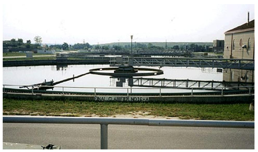
Secondary clarifiers are used to settle the mixed liquor solids.
