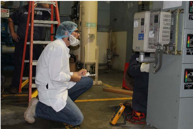
Keith Striby confirms proper placement of monitoring equipment and data loggers during a recent OSU IAC assessment.
